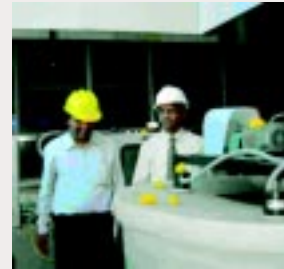
A 50 m 3 /h effluent treatment plant using the C-Tech cyclic activated sludge process at Manav Breweries Pvt. Ltd., Bulandshahr, Ghaziabad, UP.
