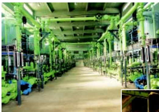
Softening and demineralisation plant and condensate polishing units for thermal power station
