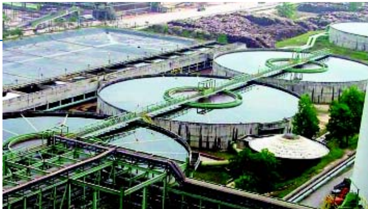
Aerial view of high rate solids contact clarifiers for pulp & paper mill
