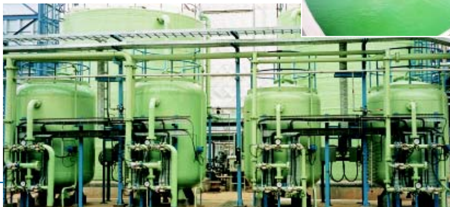
High rate solids contact clarifier and demineralisation plant for combined cycle power project
