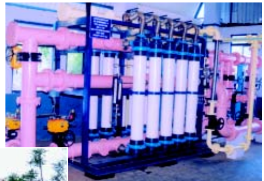
Plating effluent recycle at auto ancillary unit
