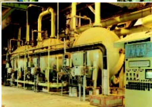
Softening and demineralisation plant and condensate polishing units for thermal power station
