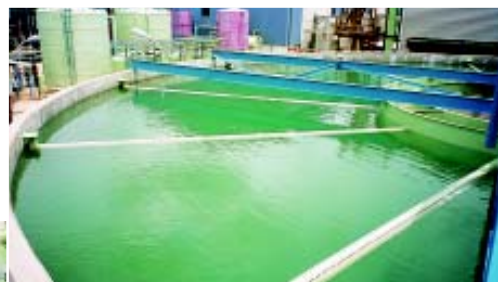
High rate solids contact clarifier and demineralisation plant for combined cycle power project
