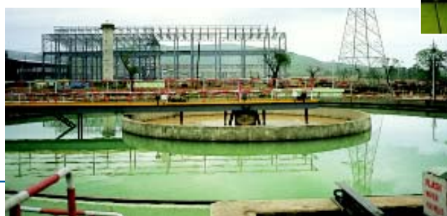
Pretreatment plant for steel industry
