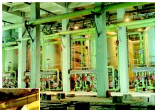
Softening and demineralisation plant and condensate polishing units for thermal power station
