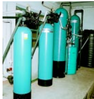
For drinking water, RO system of 0.6 m 3 /h capacity, with full pretreatment consisting of filtration, iron removal, activated carbon, softening and ultra violet sterilisation, at Defence Complex, Hastings, Kolkata.
