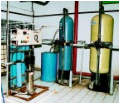
At Bengal Ambuja's City Centre Multiplex, Salt Lake, Kolkata – eastern India's largest mall, designed by Charles Correa, centralised treatment plant comprising iron removal and softening of 36 m 3 /h capacity. In addition, a drinking water RO system of 1 m 3 /h with complete pretreatment.
