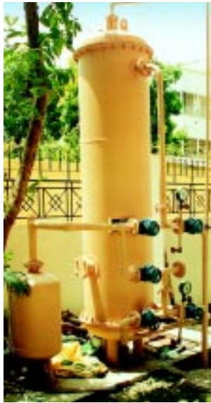
At Bengal Ambuja's City Centre Multiplex, Salt Lake, Kolkata – eastern India's largest mall, designed by Charles Correa, centralised treatment plant comprising iron removal and softening of 36 m 3 /h capacity. In addition, a drinking water RO system of 1 m 3 /h with complete pretreatment.
